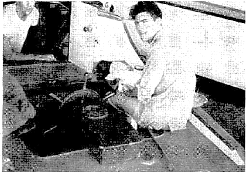
Looking aft into the Gypsy's steering compartment.
